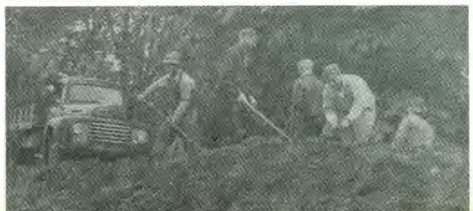
Below: Men working on the Rosedale dyke.
