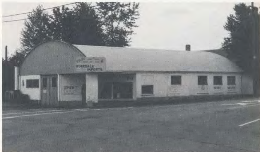
McGrath Garage Bldg. concrete walls with oval wooden trusses, constructed 1921.
