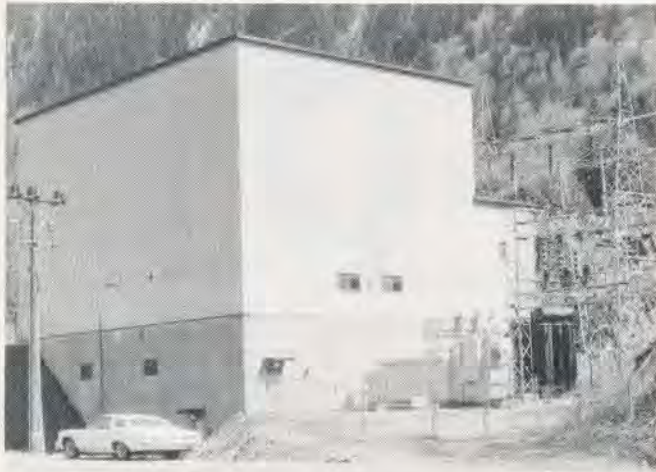
Generating Plant beside Trans Canada Highway using water from Jones Lake.
