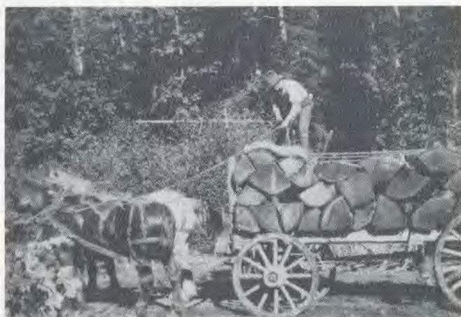
Wagon load of shingle bolts.
